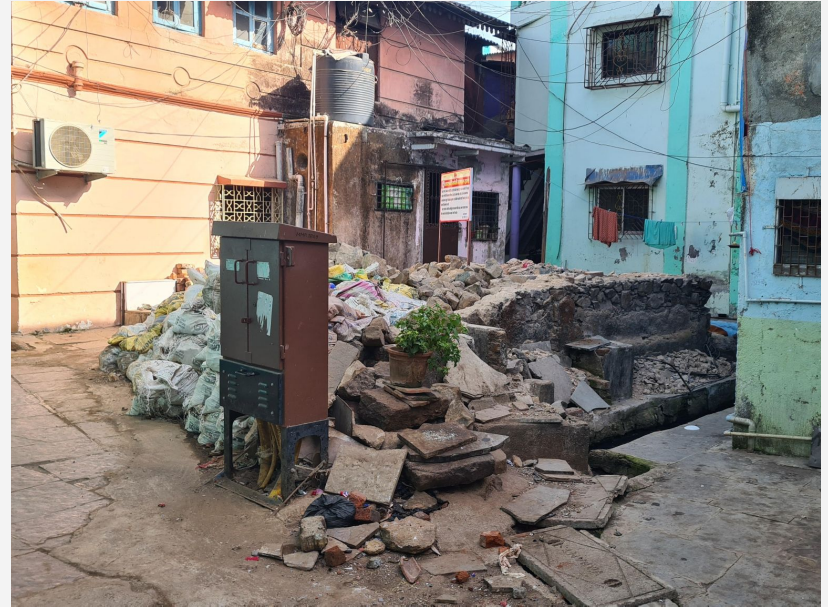
Customs House in February 2024
